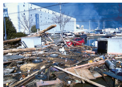
Damage from the Great East Japan Earthquake (Tohoku Branch Office)
